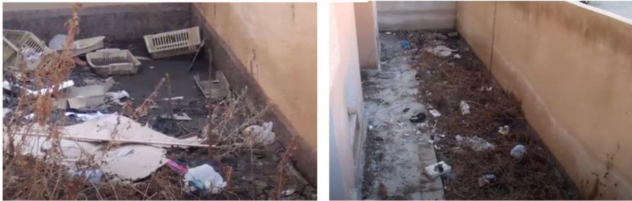
Figure 8. Accumulation of waste around the housing. (Researcher Photography 2020)
